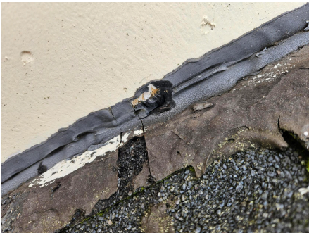
Black Roofing Mastic at Base of Tower and Roof Seam
