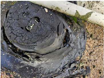
Black Roofing Mastic at Roof Penetration
